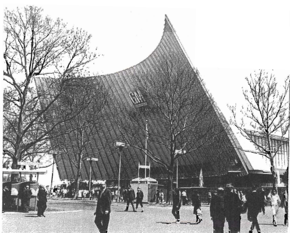
Largest building at the Fair is the General Motors Pavilion. Entering below this flaring facade, visitors see and hear the world of future.
