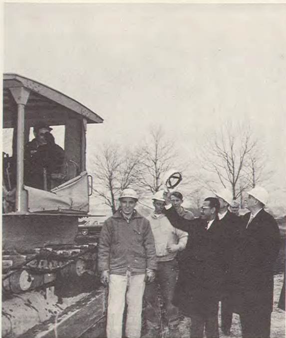
His Highness Sri Sultan Hamengku Buwono IX and Robert Moses salute the construction workers as they start excavation for the Pavilion of Indonesia.
