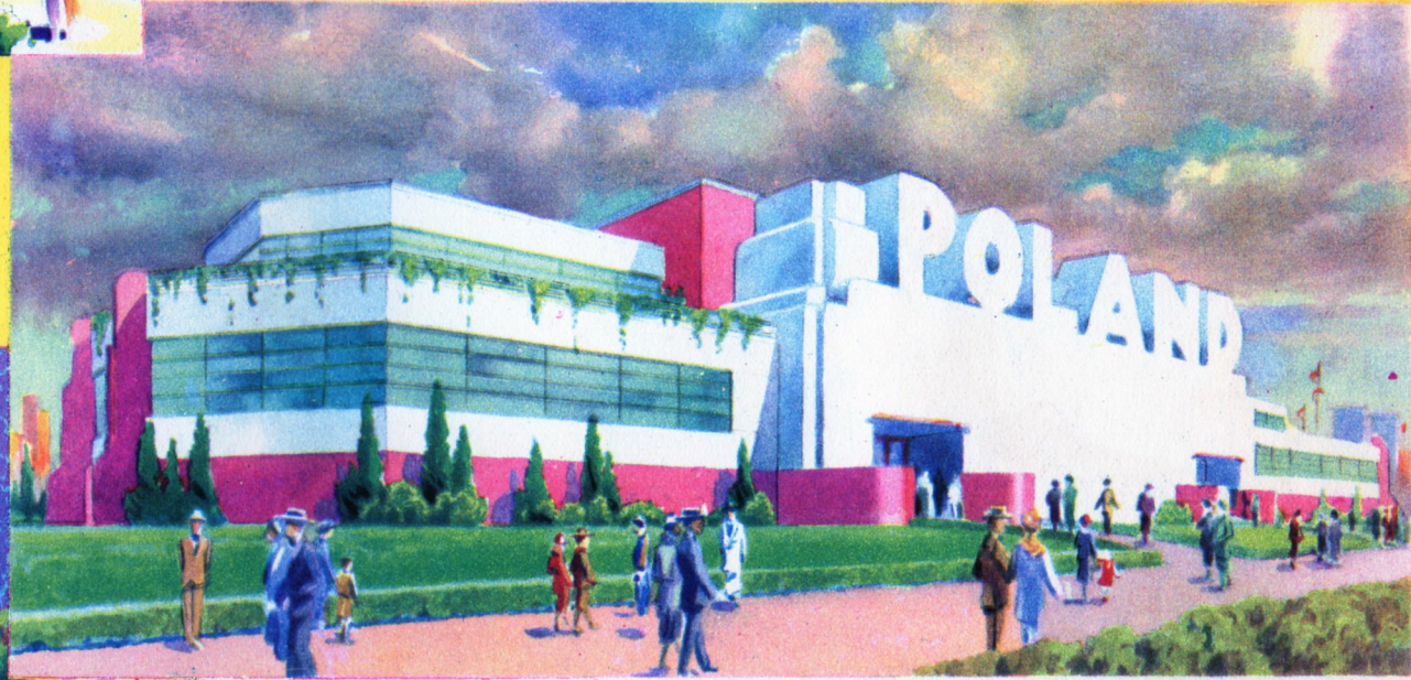
The Pavilion of new-old Poland on Northerly Island.
